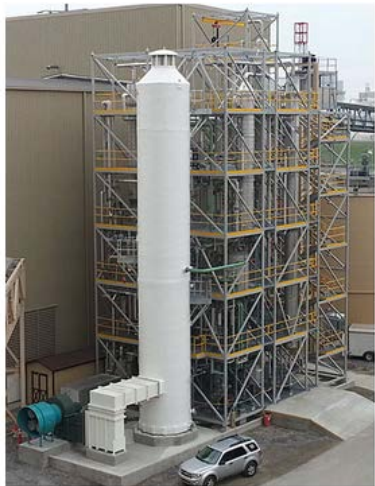
The 0.7 MWe slipstream testing facility
